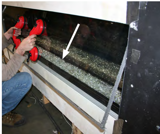
Figure 2 Sec.8 Window Removal (using glass lifting tools).
