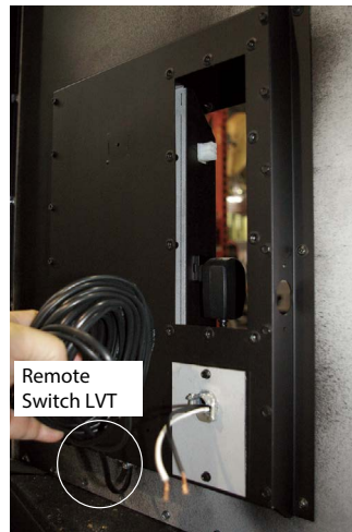
Figure 12f. Installing the Remote LVT Switch.
