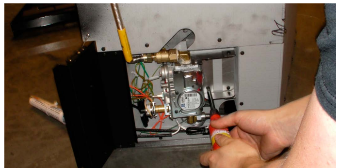
Figure 4.2 Propane conversion kit showing pilot orifice, main burner orifice,
