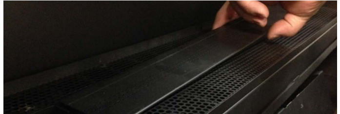
Figure 13.b Loosening the venturi
