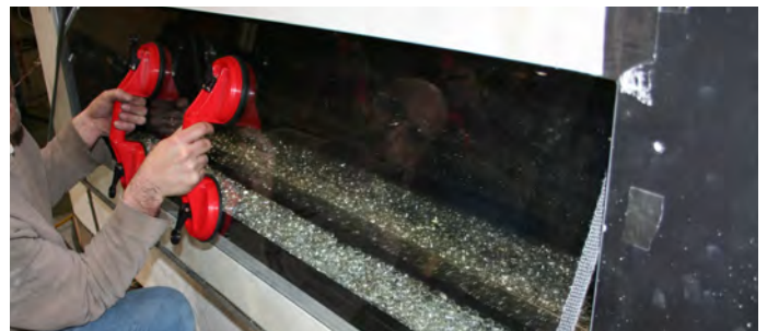
Figure 11.c Window Removal (using glass lifting tools).
