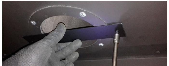
Figure 8.b.c Restrictor plate Installation
