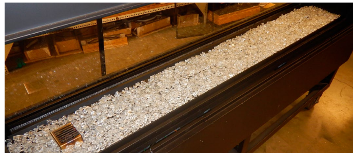
Figure 22.b Completed glass Firestone installation.
