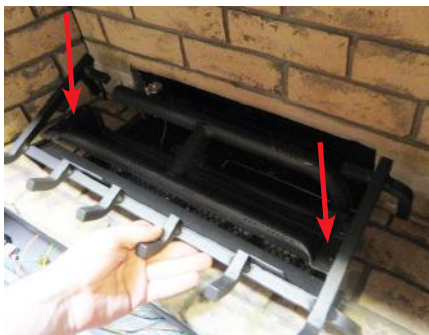
Diagram 1: Remove the left and right screws.
