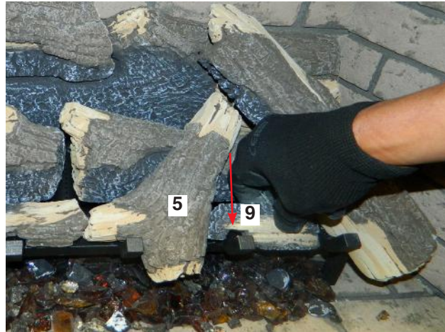
Diagram 15—Install Log 9
