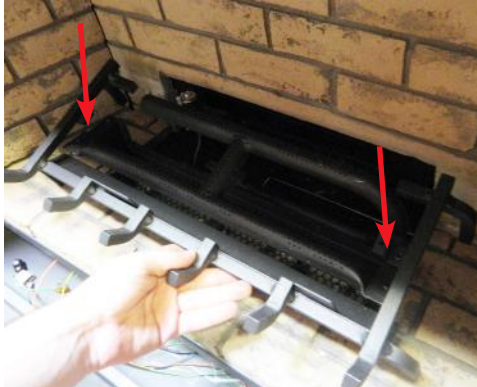
Diagram 1: Remove the left and right screws.
