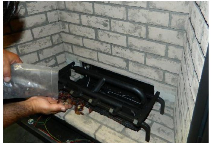
Diagram 3—Install Glass
