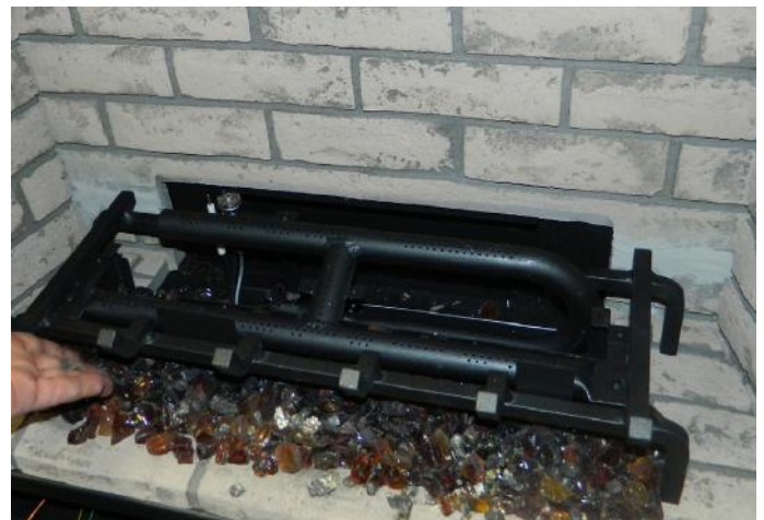
Diagram 4—Install Vermiculite + Lava
