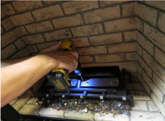
Diagram 5—Install Log support plates
