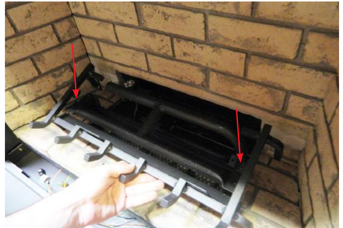
Diagram 2—Log Grate Install
