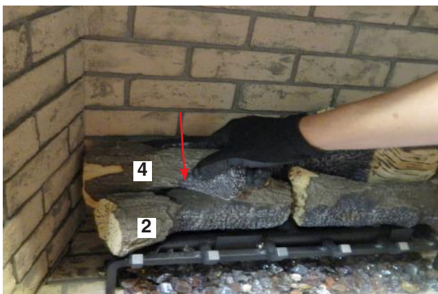
Diagram 10—Install Log 4
