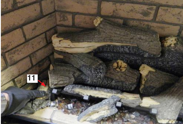
Diagram 17—Install Log 11
