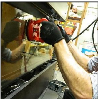
Handle glass with supplied vacuum clamps
