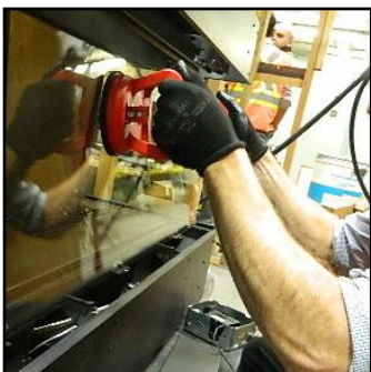
Handle glass with supplied vacuum clamps
