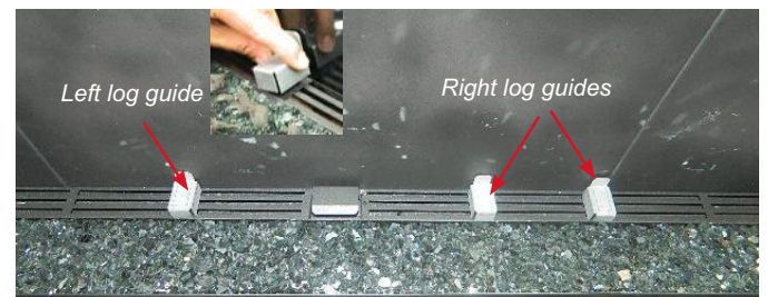
Log guides installed
