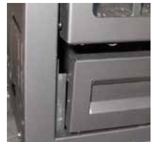
Installation of lower Flush Panel
