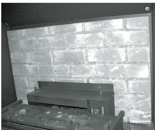
Back Panel Installed
