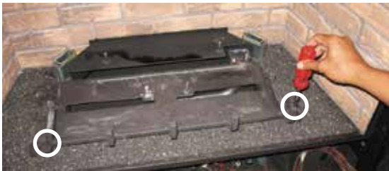
Diagram 1: Remove the left and right screws.
